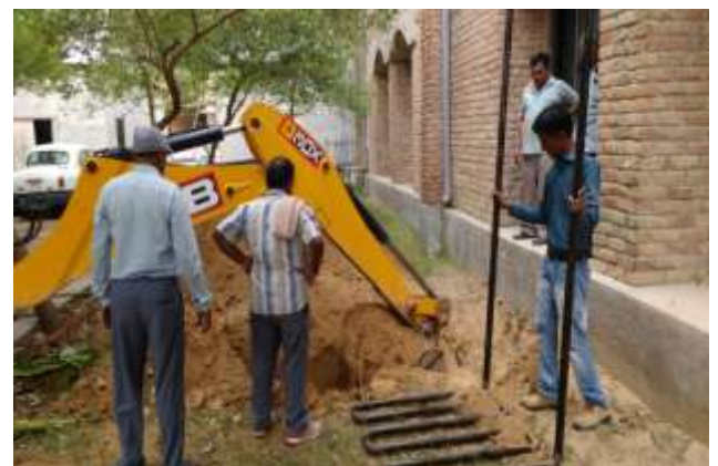
Fig. 14. Installation of Setup Using JCB Machine
