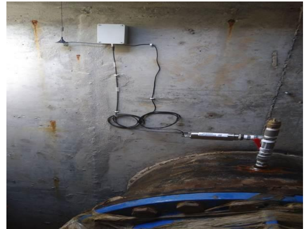
Figure 5 HiSCAN Logger with battery pack and antenna
