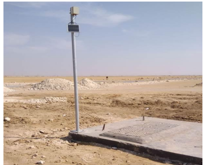
Figure 6 Installation of Alpha Data collector and solar panel on a pole near the chamber.
