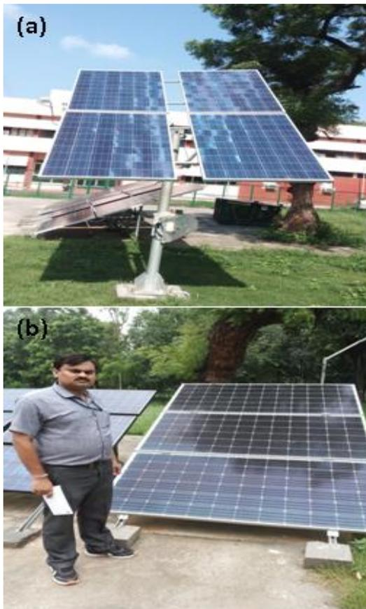
Fig. 5: (a) Rotating solar panel of 1 Kw with one LDR (dual axis) (b) Static solar panel of 1 Kw installed at CSIR-NPL, New Delhi
